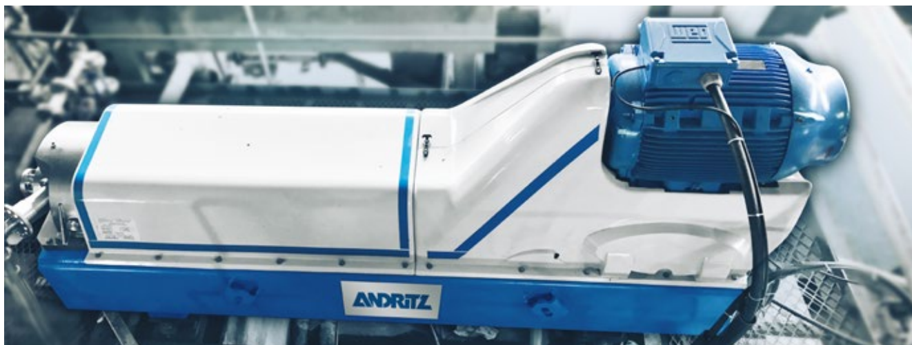
An ANDRITZ decanter centrifuge F5000, installed at a mill in Malaysia
